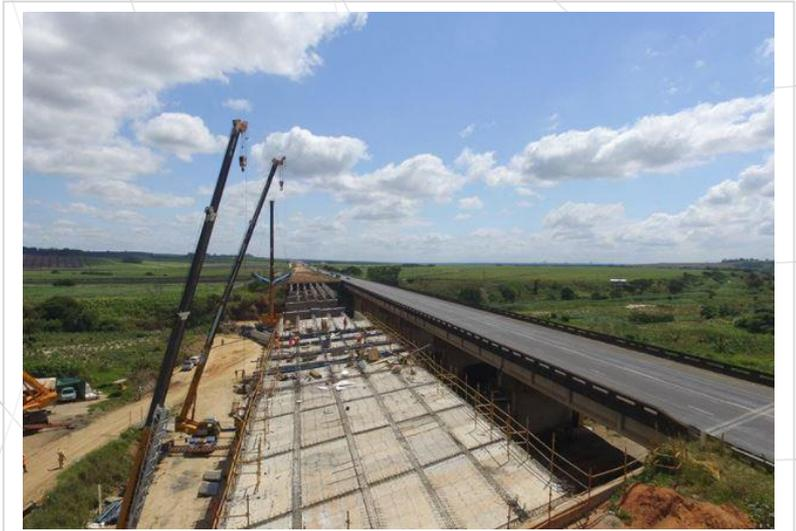
6. **UMhlathuze Rail Bridge**, which is a single-span precast post-tensioned structure. It is a type-M beam and slab bridge with closed face abutments and asphaltic plug-type joints. Its abutments are mechanically stabilised earth walls with a reinforced concrete impact wall in front. Of similar construction was the **Empangeni Rail Bridge** over the Empangeni-Richards Bay railway, which has a central pier of three wall type columns supported on 18 friction grip CFA piles 13 metres deep.
