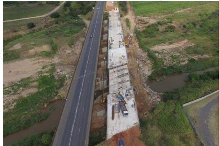
washed into the river during the bridge building stages, thereby preserving water quality and river life. The platform on the south-west side of the river gave access to pier 1, while the second platform from the north-east provided access to piers 2 and 3.
